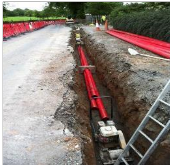
Figure 3 - 110kV Underground Duct Installation
