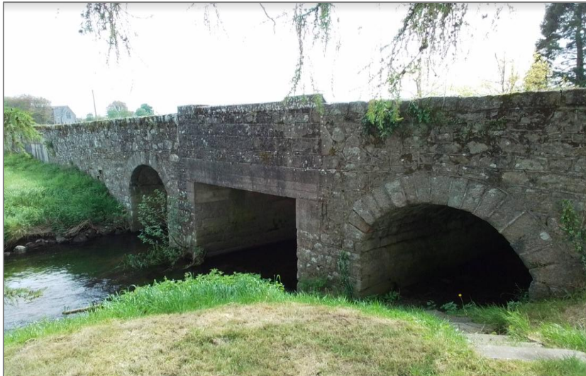
Figure 17 - Bridge 1 Rathoe Bridge
