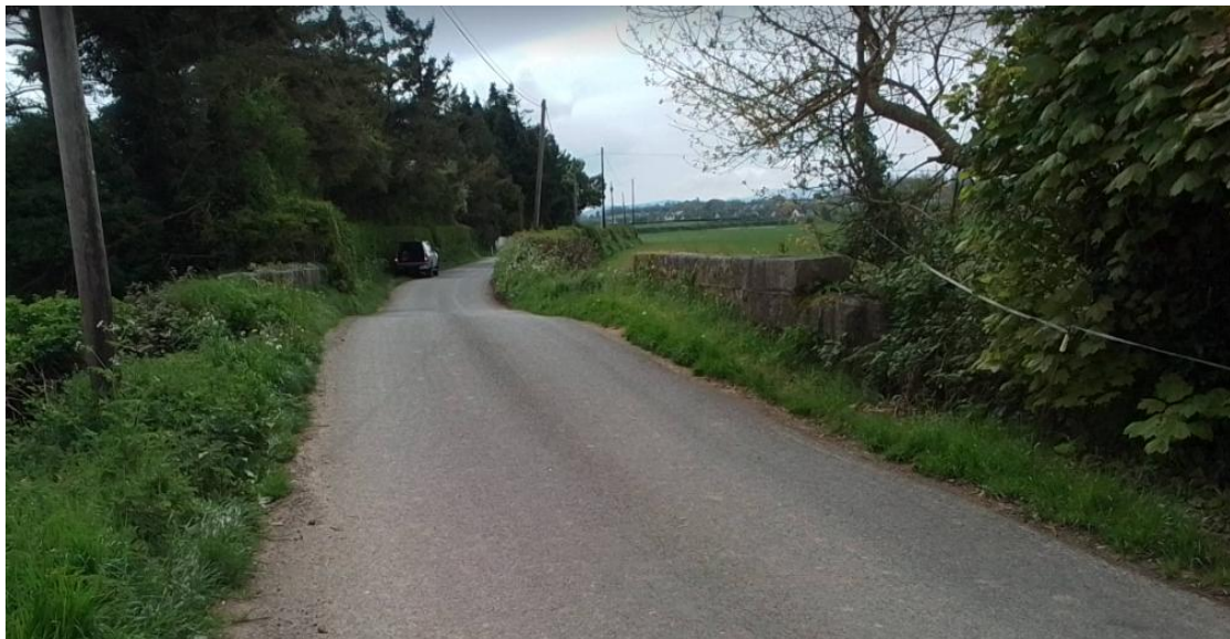
Figure 18 - Bridge 2 on River Burren Tributary
