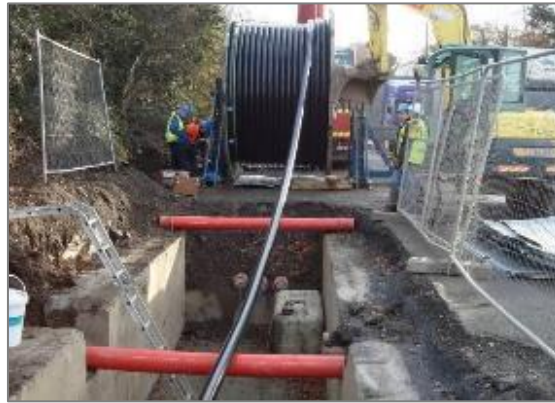
Figure 13 - HV cable pulling procedure (Typical drum set-up)
