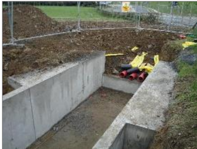
Figure 11 - Completed joint bay prior to cable installation (in-situ)
