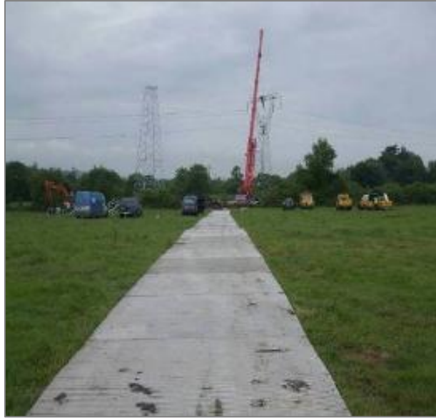
Figure 22 - Temporary Aluminium Panel Tracks
